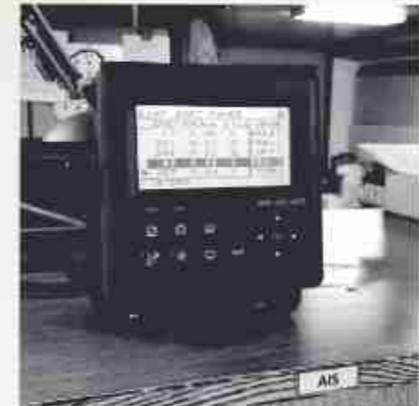
Backup Systems Installation
